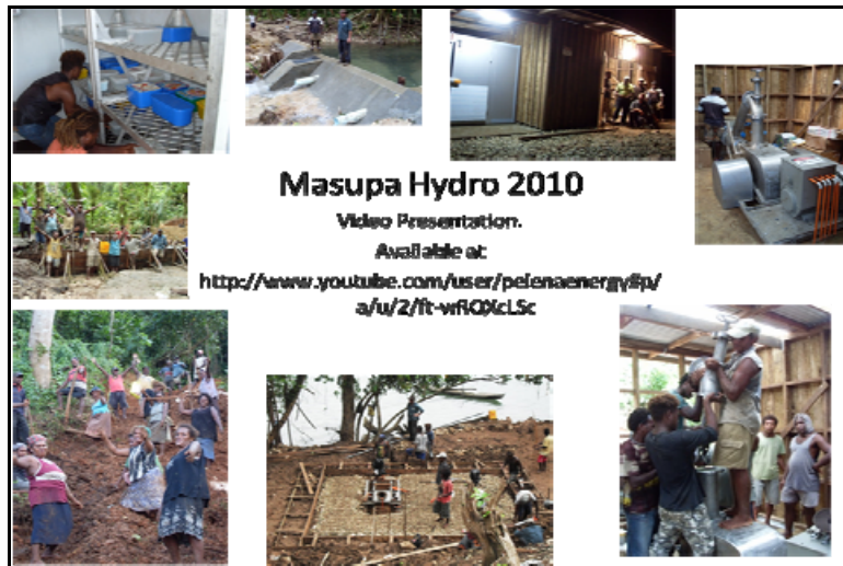
Fig 2: Pictures from the Construction of Masupa Hydro, Jan-Feb 2010
